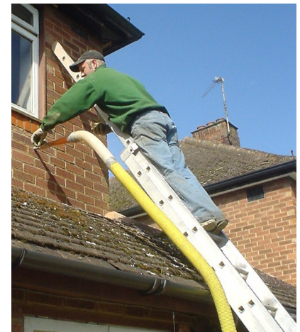
Figure 21.5. Cavity-wall insulation going in.
