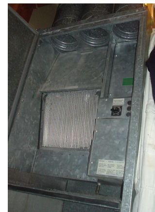
Figure E.11. The Heatkeeper's heat-exchanger.
