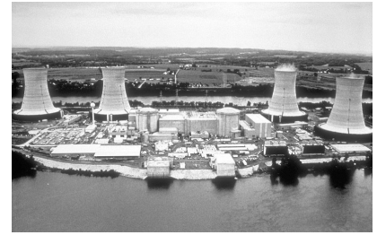
Figure 24.4. Three Mile Island nuclear power plant.
