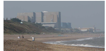
Figure 24.9. Sizewell's power stations. Sizewell A, in the foreground, had a capacity of 420 MW, and was shut down at the end of 2006. Sizewell B, behind, has a capacity of 1.2 GW. Photo by William Connolley.
