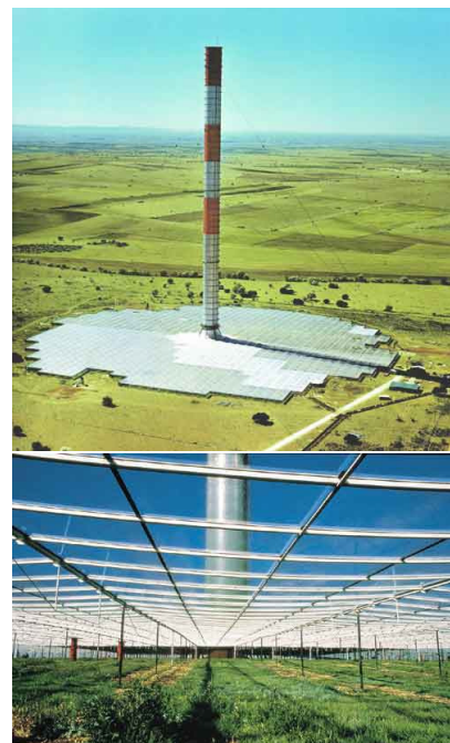
Figure 25.10. The Manzanares prototype solar chimney. Photos from solarmillennium.de .
