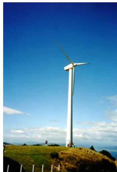
Figure B.3. The Brooklyn windmill above Wellington, New Zealand, with people providing a scale at the base. On a breezy day, this windmill was producing 60 kW, (1400 kWh per day). Photo by Philip Banks.
